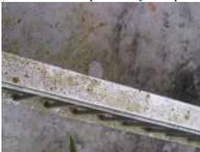
Stainless Steel Railing
